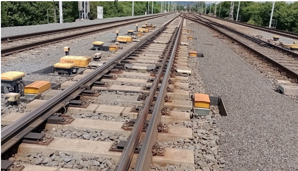
Fig. 2. Turnout switch on a railway line in the Czech Republic
