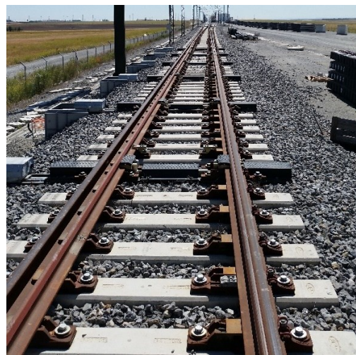
Fig. 1. Turnout for high speed trains in Spain [Source: Authors library]
