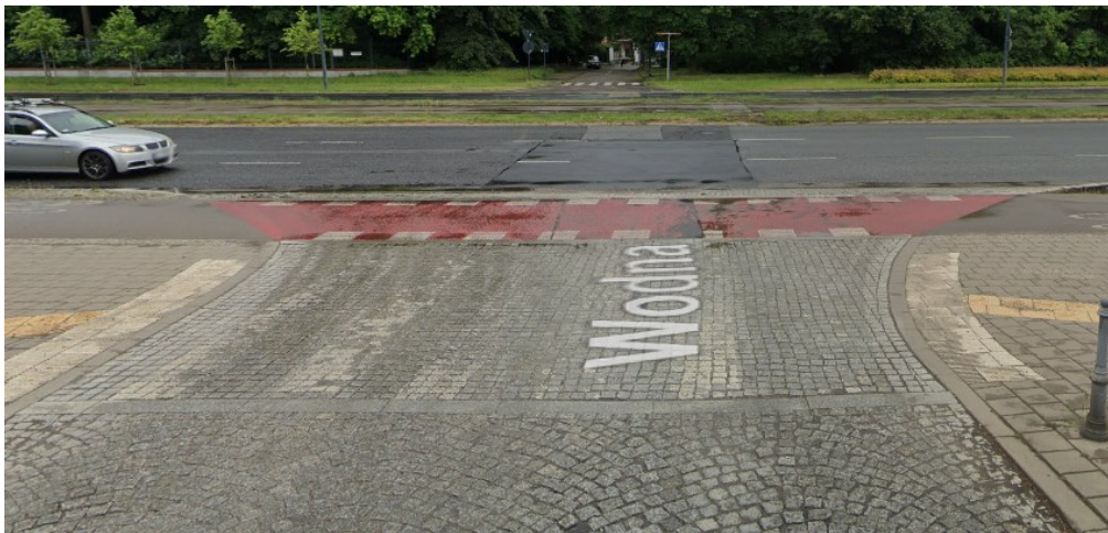
Fig. 2. A bicycle crossing that is designated on the road that the driver changing direction is leaving [23]
