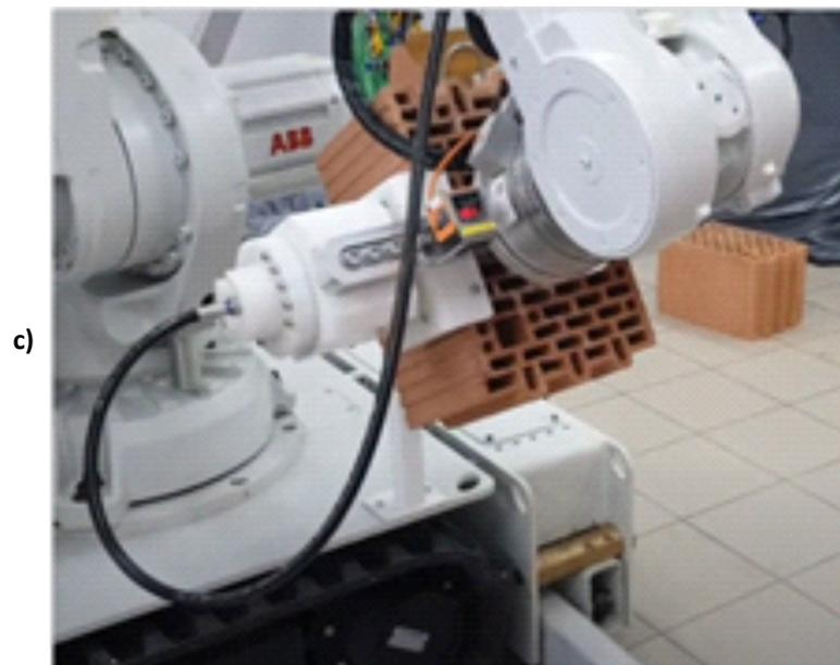
Fig. 14.c View of the bricklaying process on a partition wall: apply mortar to the bricks [16]
