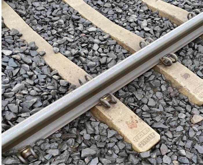
**Fig. 3. SB fastening system in PKP PLK tracks**
