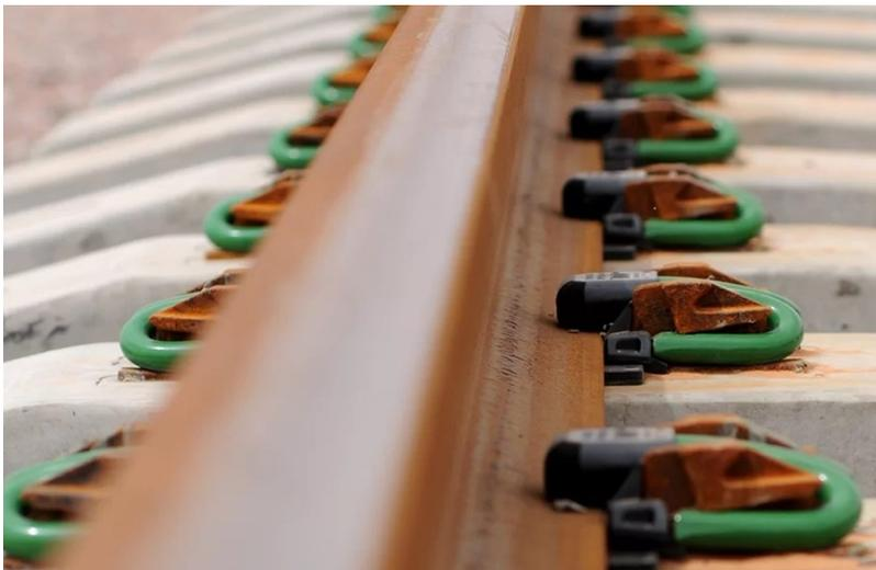
**Fig. 2. Fastening system type Fast Clip [9]**
