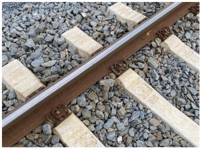
Fig. 1. Fastening systems W14 on B70 prestressed sleepers W14 in Czech Republic
