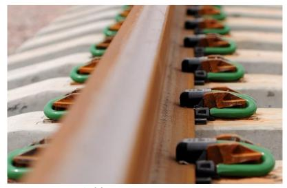
Fig. 2. Fastening system type Fast Clip [9]
