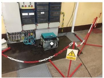
Fig. 24. Place and method of connecting the power quality analyzer Memobox 800
