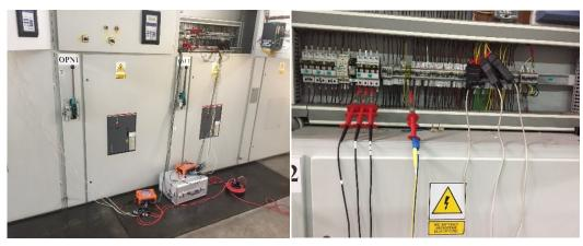
Fig. 2. Connecting PQM analyzers to measurement circuits
